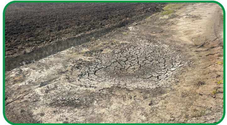
Figure 1: poorly structured soils with low permeability in Hanford, CA.
